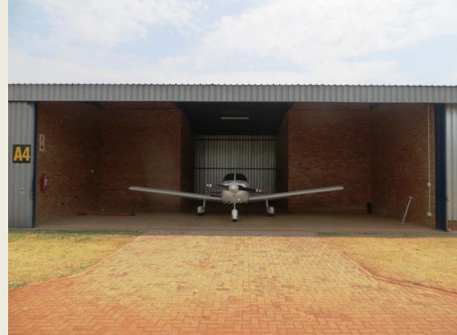
T-Hangar at FAWB – R450 000 exc. VAT
